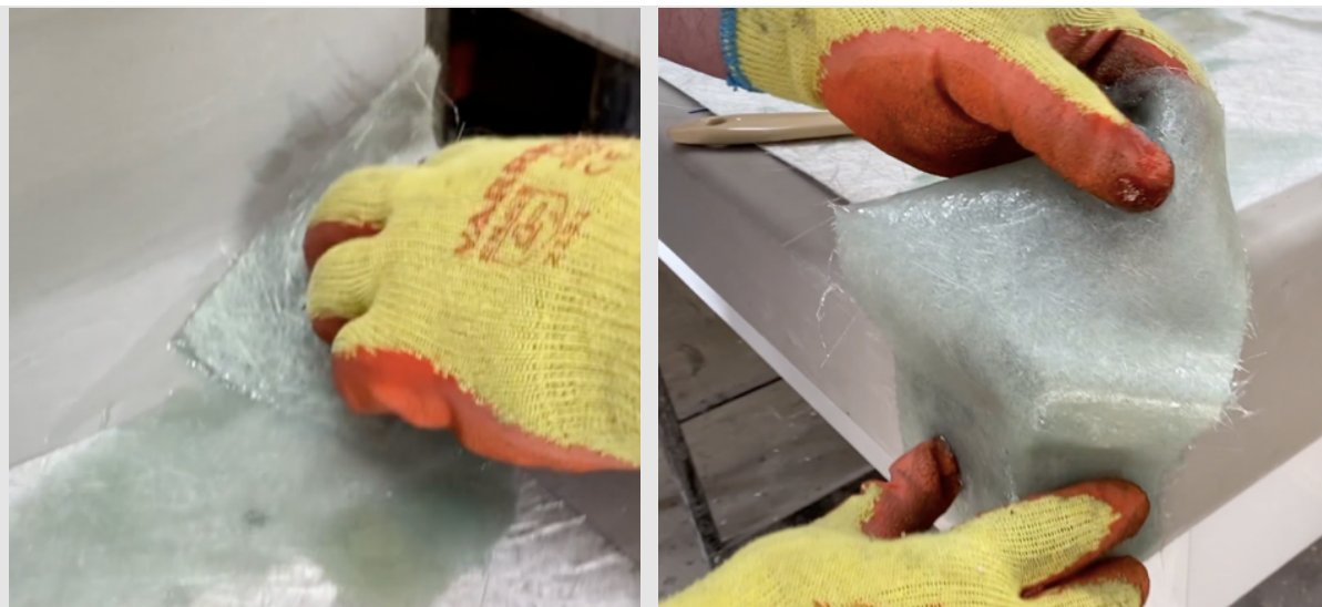
Pre-cut sections of resin-soaked matting being positioned onto corners
