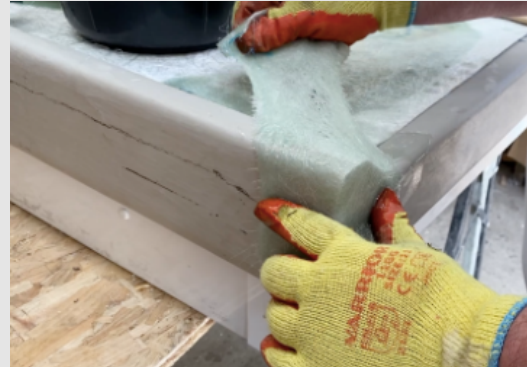
Pre-cut sections of resin-soaked matting being stretched across the corners
