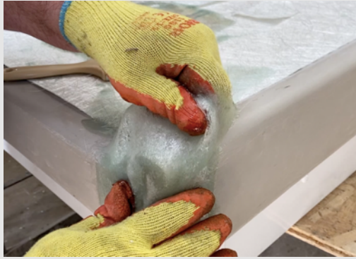
Pre-cut sections of resin-soaked matting being stretched across the corners
