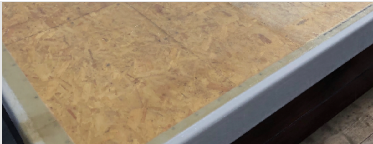
Picture of laminated flat roof post application and pre-curing
