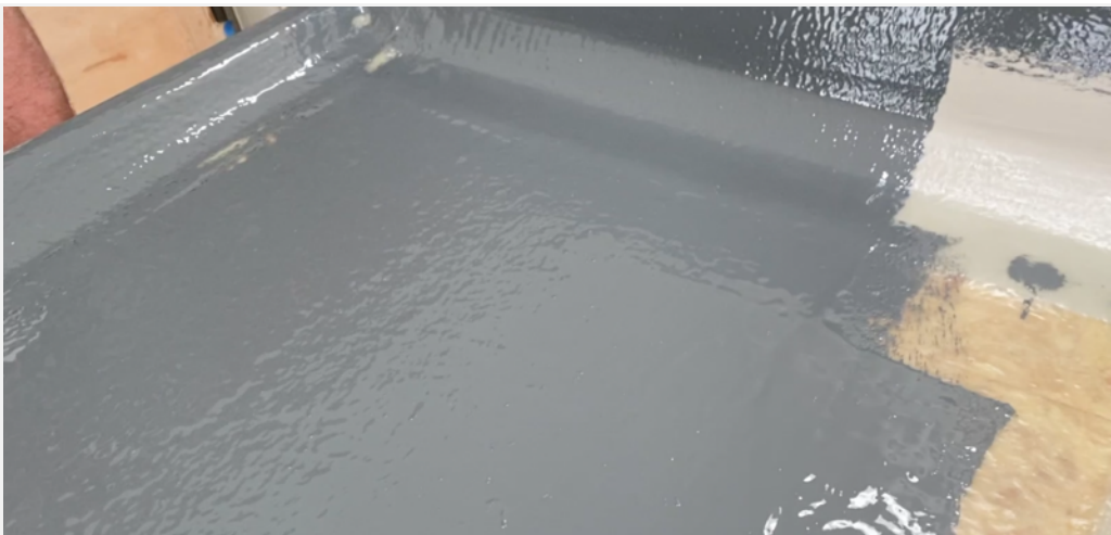
Topcoat coverage should be thin and consistent across the surface
